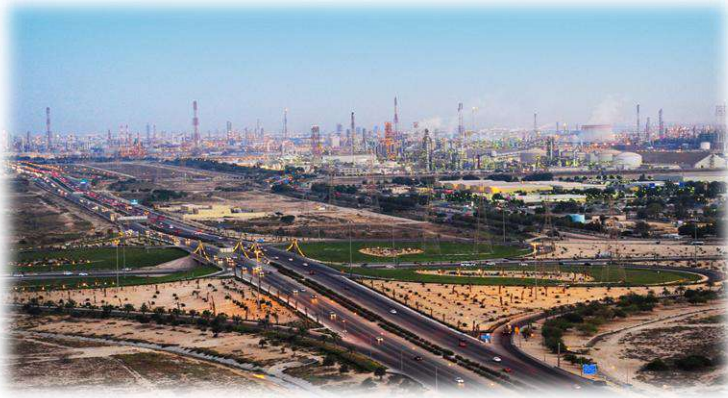
Project: Yanbu PS2 Expansion Project Main contractor: Ektebarat Engineering Contracting Co. Client: SEC Scope of Work : Civil works
