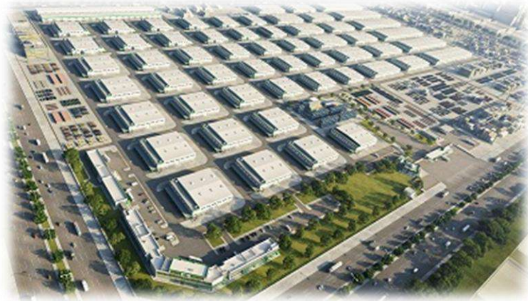
Project: MSSD Shops Expansion Project Main contractor: MASCO General Contracting Client: ARAMCO Scope of Work : Civil works
