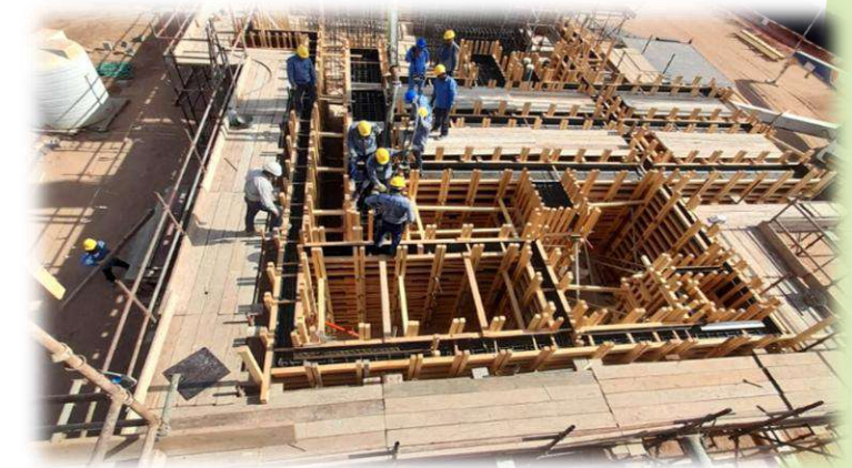
Project: Wadi Al-Dawaser - Expansion project Main contractor: Ektebarat Engineering Contracting Co. Client: SEC Scope of Work : Civil works
