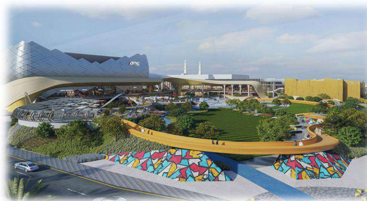
Location: Madinah Main contractor: Nicolas-NN GROUP Client: SEVEN Scope of Work : HVAC works
